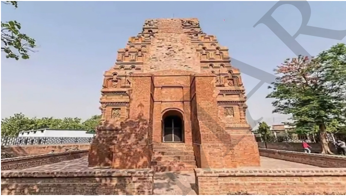
Bhitargaon Temple, Kanpur, Uttar Pradesh
