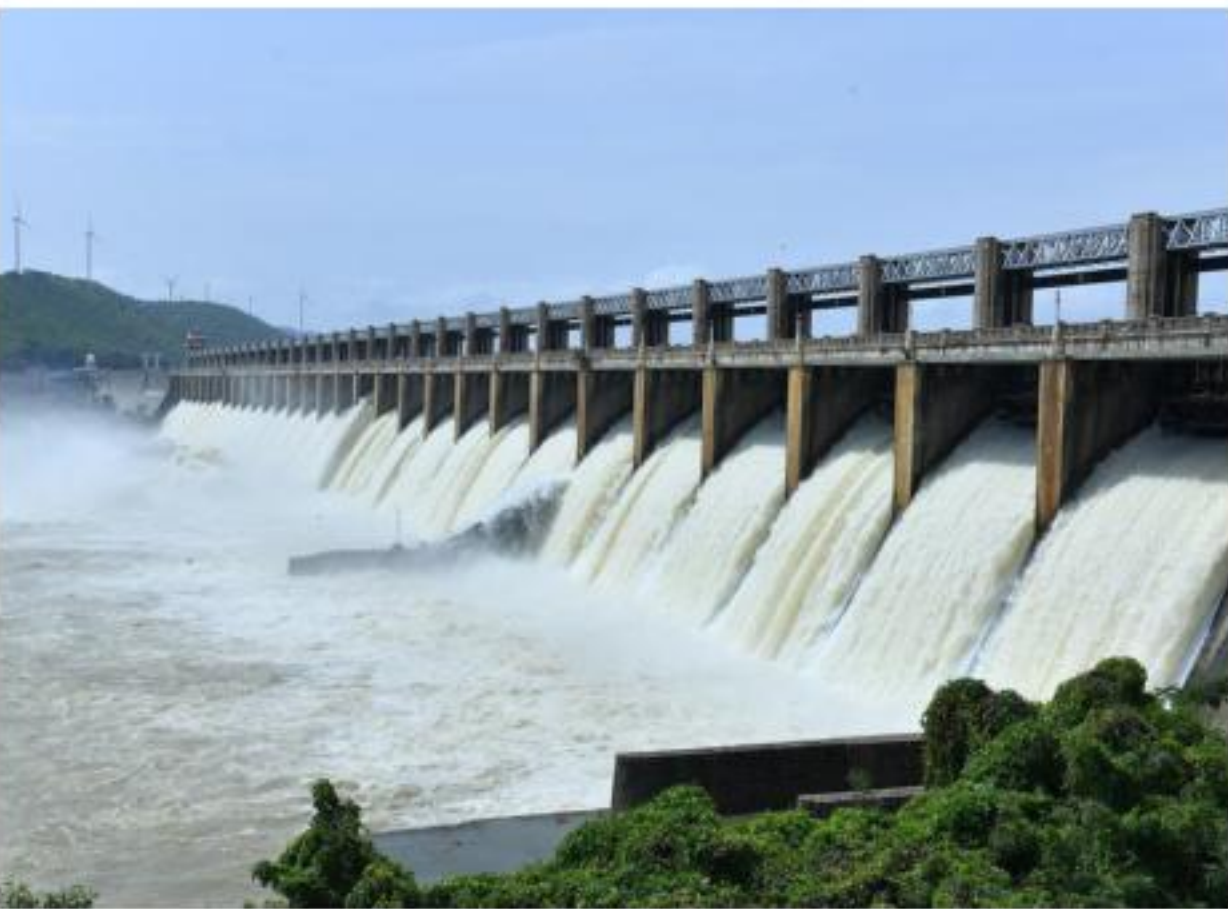
Water wastage: Officials had to increase discharge to 98,000 cusecs by opening all 32 gates at the Tungabhadra reservoir to reduce pressure on the broken gate. SRIDHAR KAVALI
